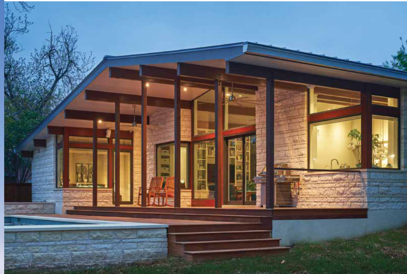
(TOP) THE FULL-SCALE, MID-CENTURY REMODEL OF THIS 1950S-ERA HOME INCLUDED RAISING THE ROOF, ALONG WITH AN ADDITION AND A PORCH. THE HOME'S NEW LOOK IS DESIGNED TO FIT IN WITH THE 1950S RANCH HOMES IN THE NEIGHBORHOOD. (PHOTO BY LEONID FURMANSKY)
