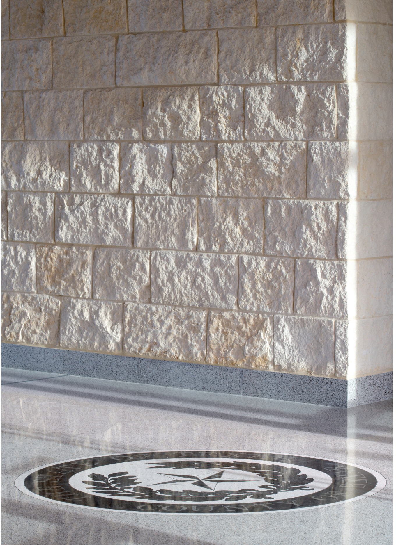
"For the outside, limestone served as the literal foundation for Bexar County Public Works and also the inspiration for the rest of the exteriors materials pallet," said Angel Garcia, of Marmon Mok Architects. "Complementing the exterior limestone, the outside also features weathering steel, zinc metal panels, glass and wood composite accents. For the interiors, the same limestone was used."
