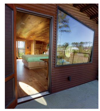
longleaf pine. Using Cor-Ten steel, also known as weathering steel, eliminates the need for painting; as the product ages and is exposed to the elements, it develops a stable, rusted patina. A deck overlooks the growing young forest, and a simple spiral labyrinth — an extension of a stone archway over the walking path — adds texture and intrigue to the landscape below.
