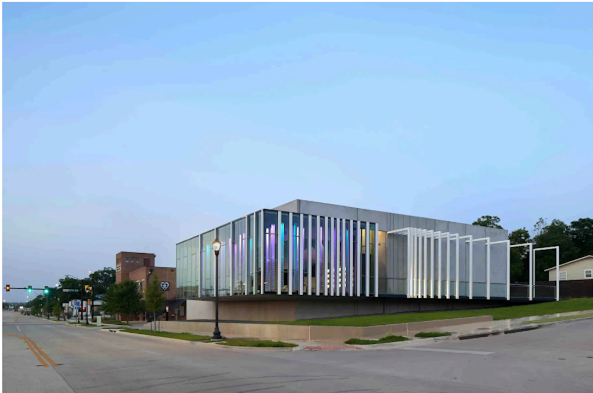
The design of the office takes advantage of the location.
