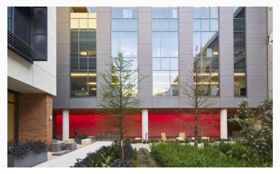
To meet LEED Gold standards, architects wrapped the building with a highly insulating envelope punctuated with fullheight windows and wove biophilic design elements throughout the interior. Daylight responsive LEDs and an HVAC system that draws chilled water from Austin Energy's Mueller District Energy System help to further reduce the building's energy footprint.
