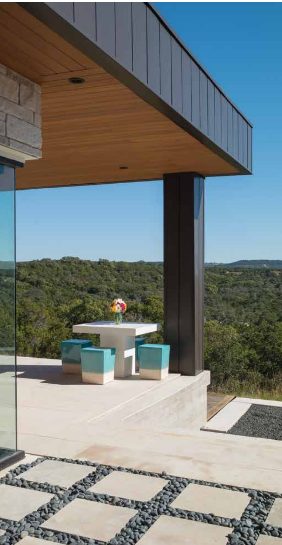
A covered patio is located right off the living room.
